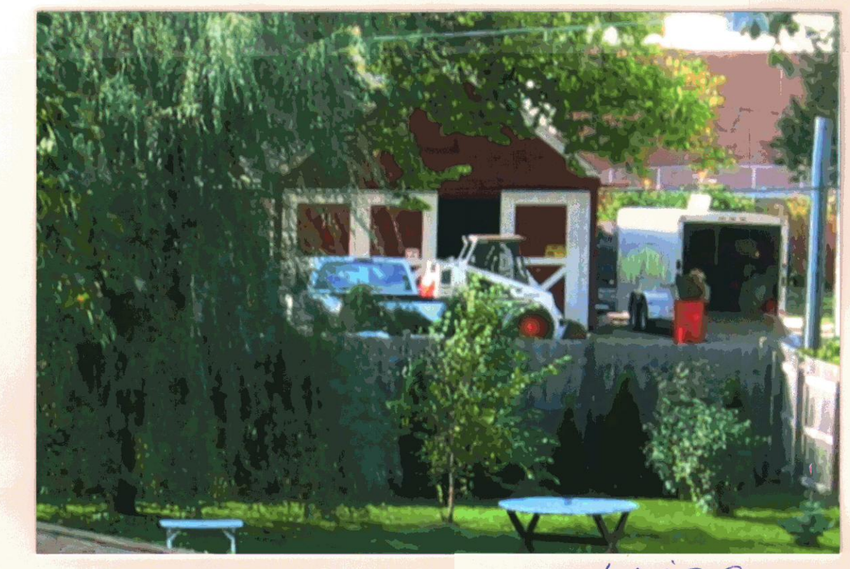
lots of activity & noise. Moving debris around with bobcat
