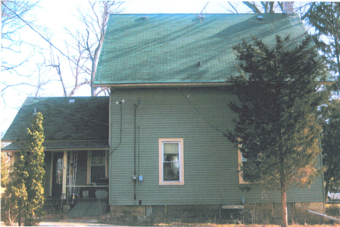
Photo #2– West Elevation
