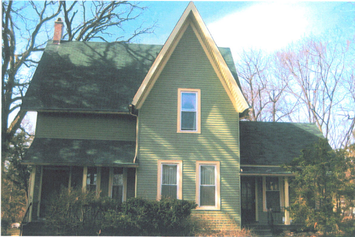
Photo #1 – East Elevation
