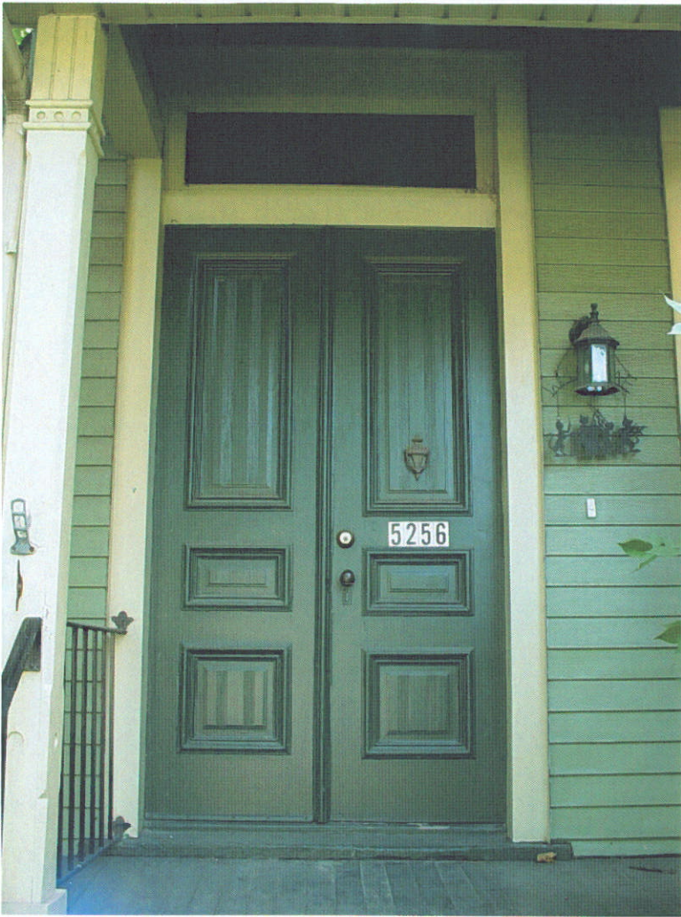
Photo #5 – East Elevation – Double door
