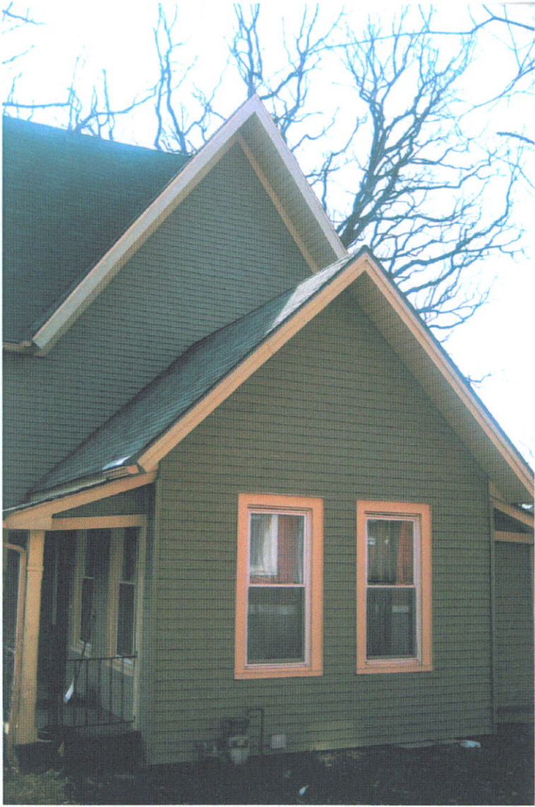
Photo #4 – North Elevation
