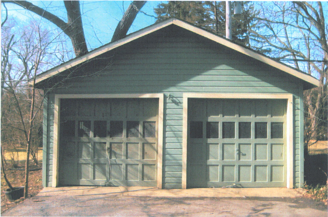
Photo #6 – East Elevation - Garage
