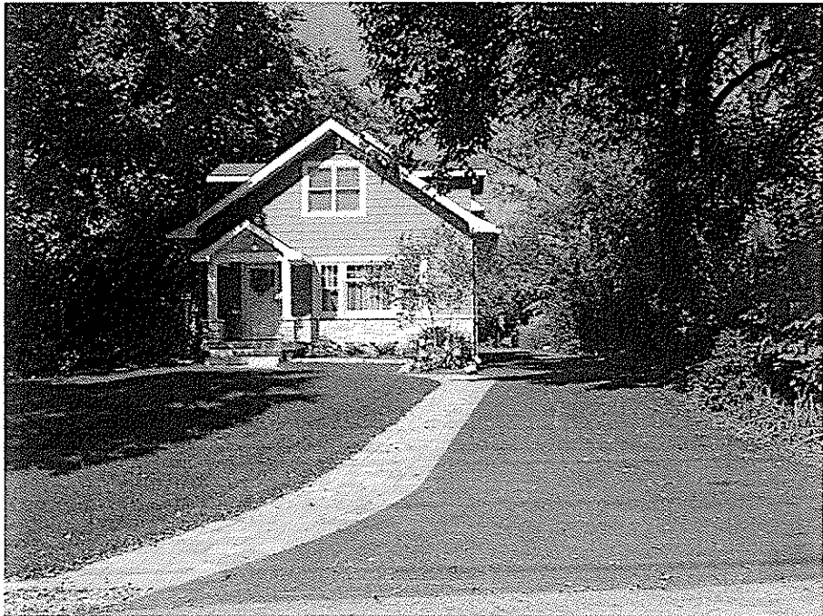
064 – 2340 COLLEGE – MAJOR RENOVATION
