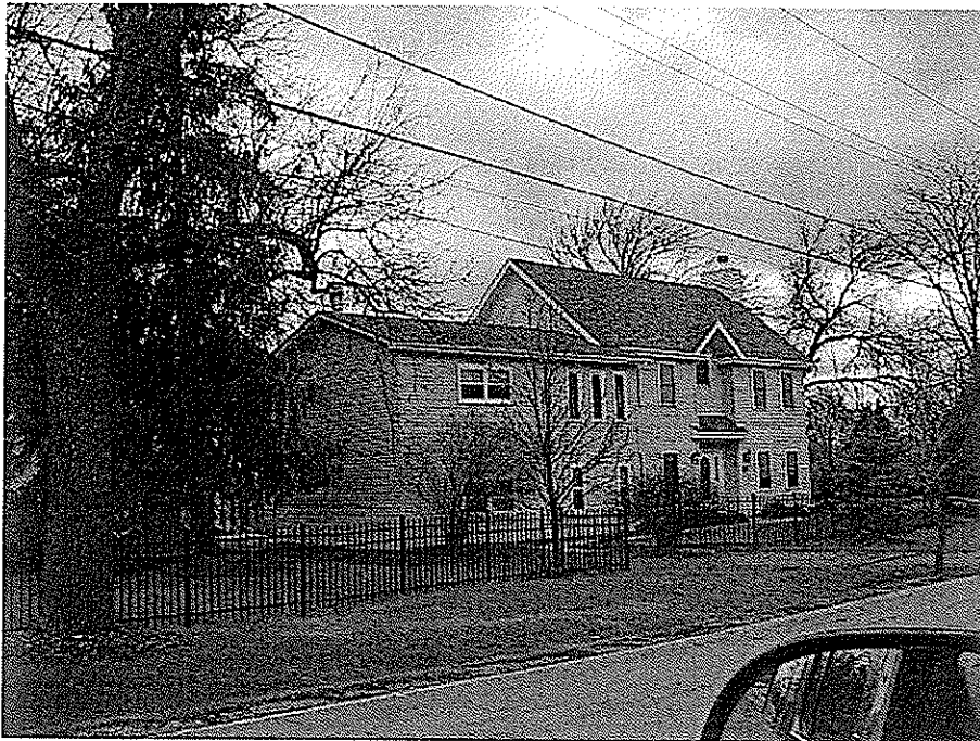
034 – 5602 ELINOR – MAJOR RENOVATION
