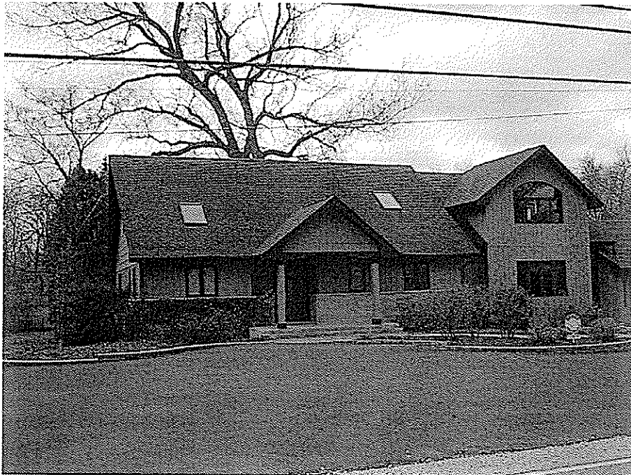
018 – 2333 COLLEGE – MAJOR RENOVATION
