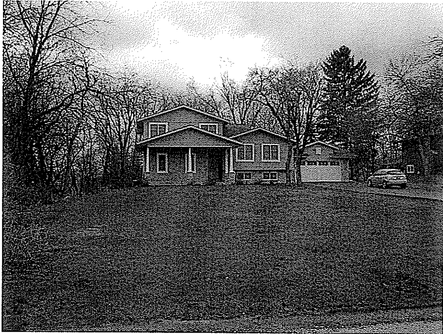
009 – 5858 CHASE – MAJOR RENOVATION
