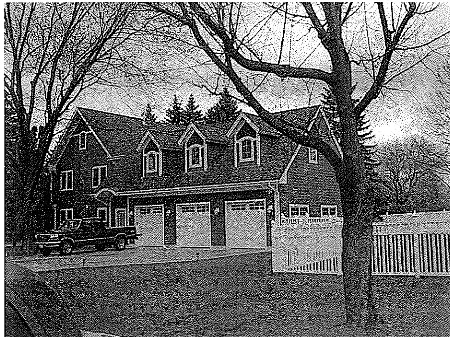
040 – 5617 KATRINE – MAJOR RENOVATION
