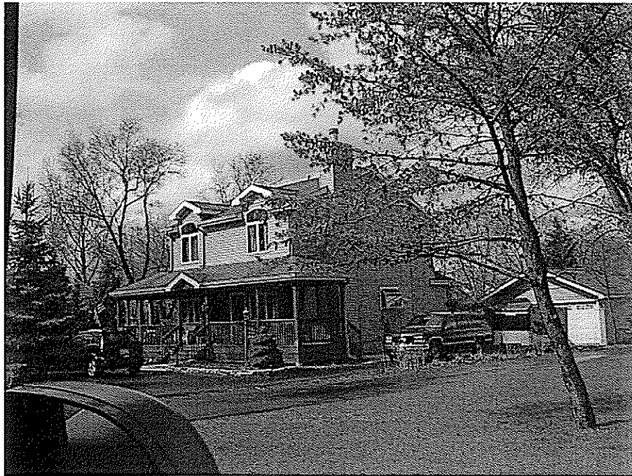
044 – 5612 KATRINE – MAJOR RENOVATION
