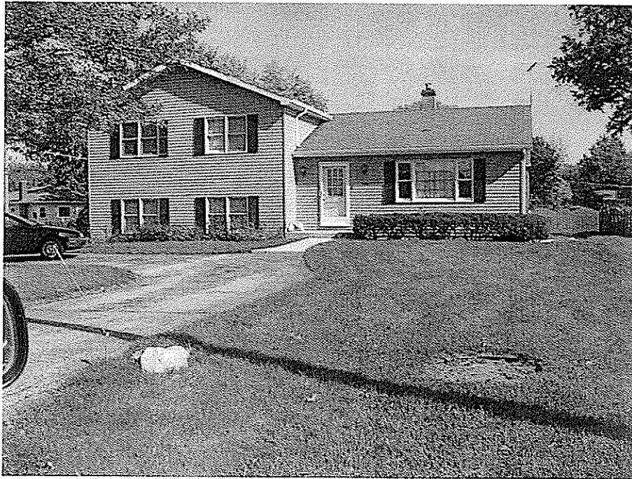
058 – 5603 KATRINE – MAJOR RENOVATION
