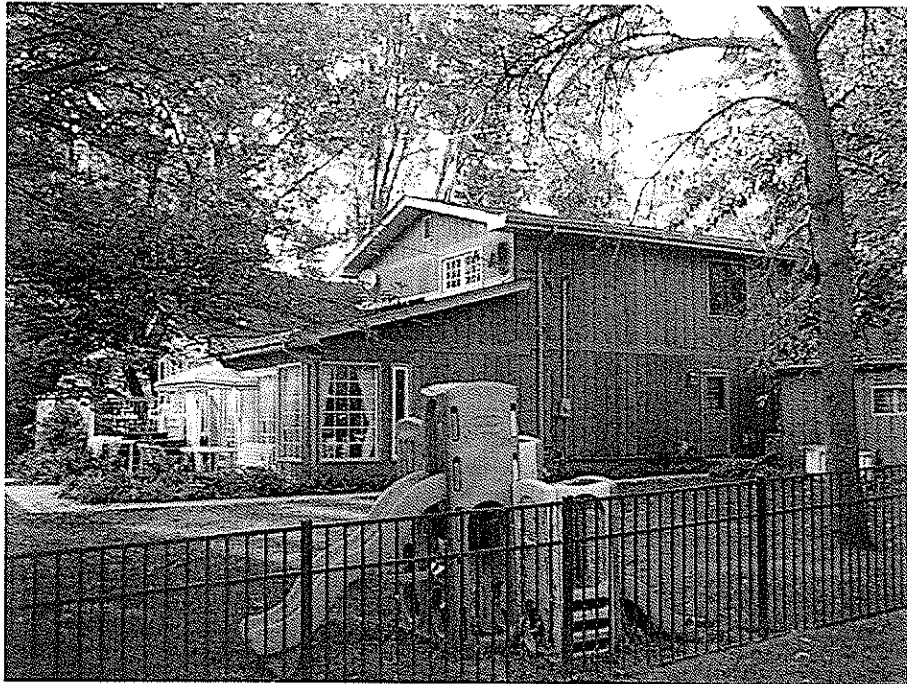
061 – 2505 COLLEGE – MAJOR RENOVATION
