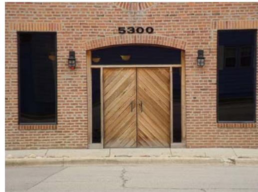
Fig. 10: Opaque windows and windows which do not make up the majority of the storefront should be avoided.
