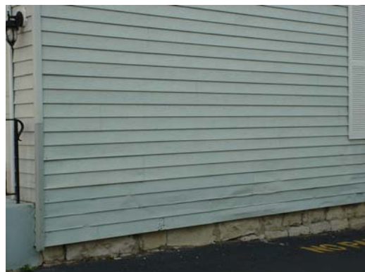
Fig. 36: Vinyl and aluminum siding should not be used to cover historic building materials
