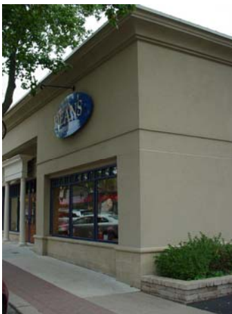
Fig. 17: Materials such as EIFS can be used effectively as an accent. However, it should be avoided as a primary material on first floor
