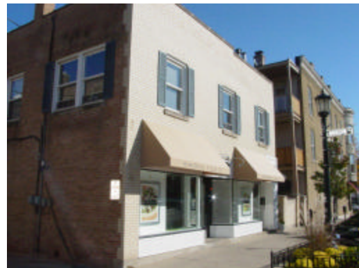
Fig. 40: It is important to provide details at the top of buildings. In this example, the parapet does not have any detail or cornice. Buildings without detail at the top should be avoided
