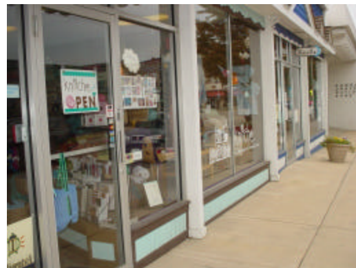
Fig. 8: Encouraged: knee walls and windows which make up a majority of the storefront
