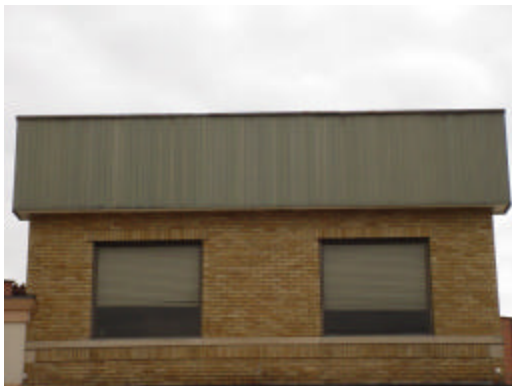
Fig. 39: Cornices should have detailing and should be in scale with the rest of the building. New cornices should not cover original features.
