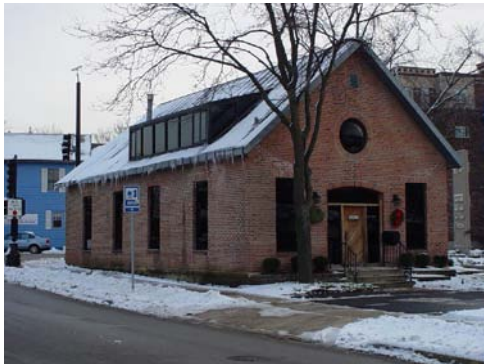
5300 Main St – Sucher Blacksmith House ◆
