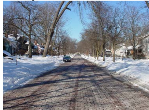
4700-5000 Middaugh Ave – Brick Street ◆
