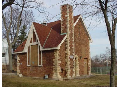
5324 Park Ave – Old Pump House +
