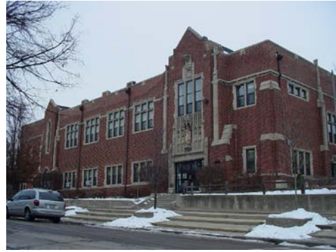
4832 Highland Ave – St. Joseph School +
