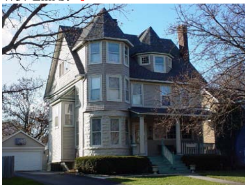
5228 Fairmount Ave – Sterling North House ◆
