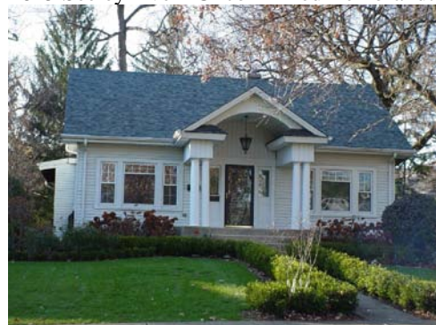
4916 Seeley Ave – Unconfirmed Crescent ▲
