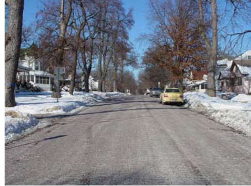
4800-4900 Saratoga Ave – Brick Street ◆
