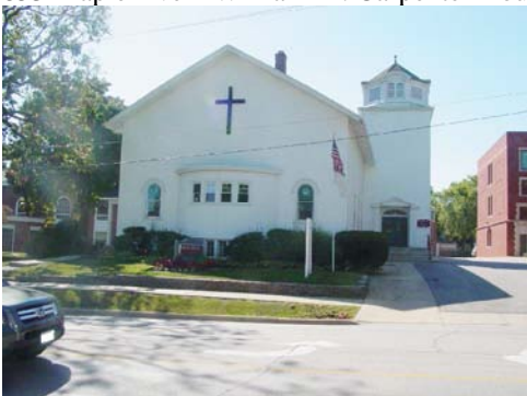
929 Maple Ave – First Baptist Church + ◆
