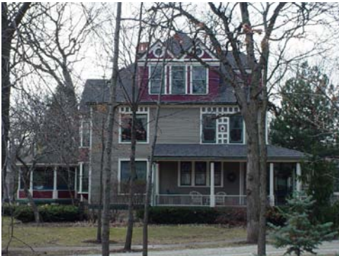
4714 Oakwood Ave – E. H. Prince Mansion +
