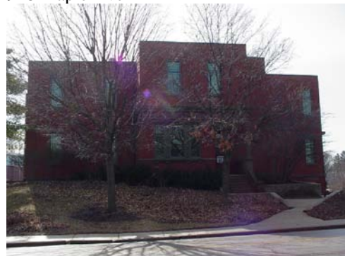
935 Maple Ave – Lincoln Center + ◆
