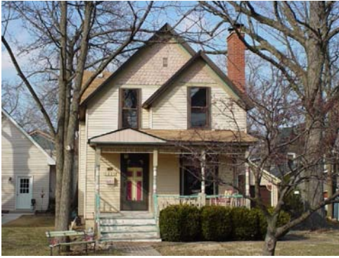
1220 Warren Ave – Lewis P. Sucher House + ◆
