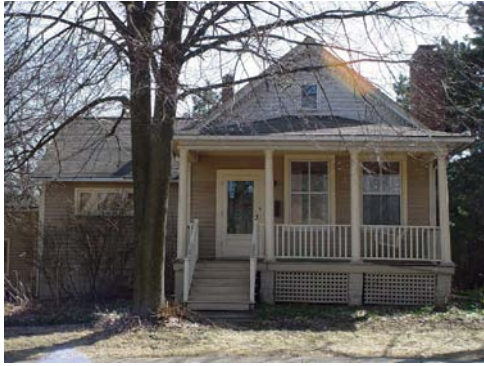
1525 Jefferson Ave – Unincorporated DG +
