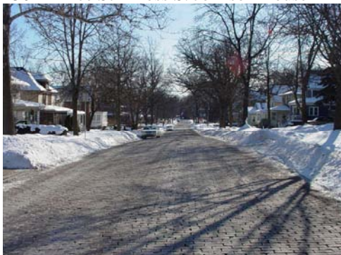
4700-4900 Prince St – Brick Street ◆
