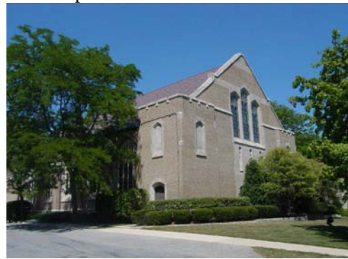
1032 Maple Ave – 1 st United Methodist Church +
