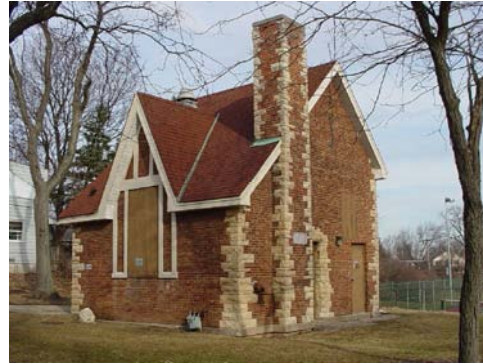
5324 Park Ave – Old Pump House +
