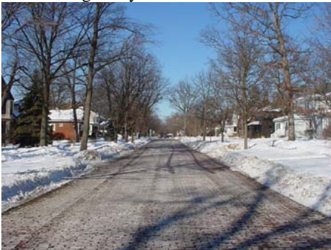
4700-5000 Oakwood Ave – Brick Street ◆
