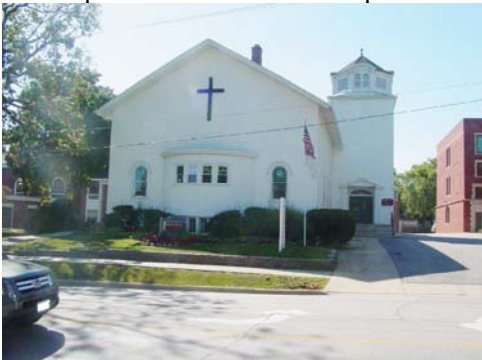
929 Maple Ave – First Baptist Church + ◆
