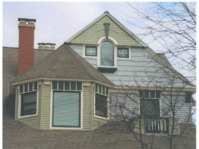
Figure 4. Second story of west facade
