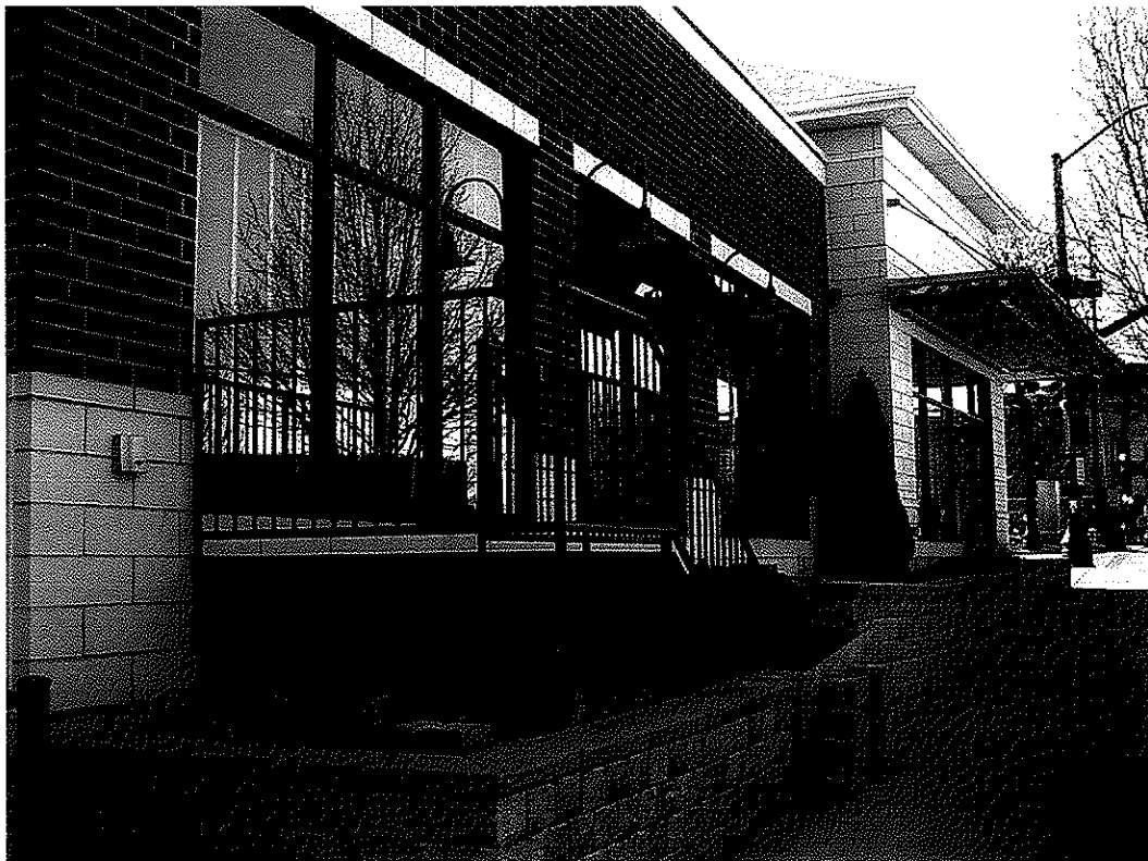
Figure 4 – West seating area looking south
