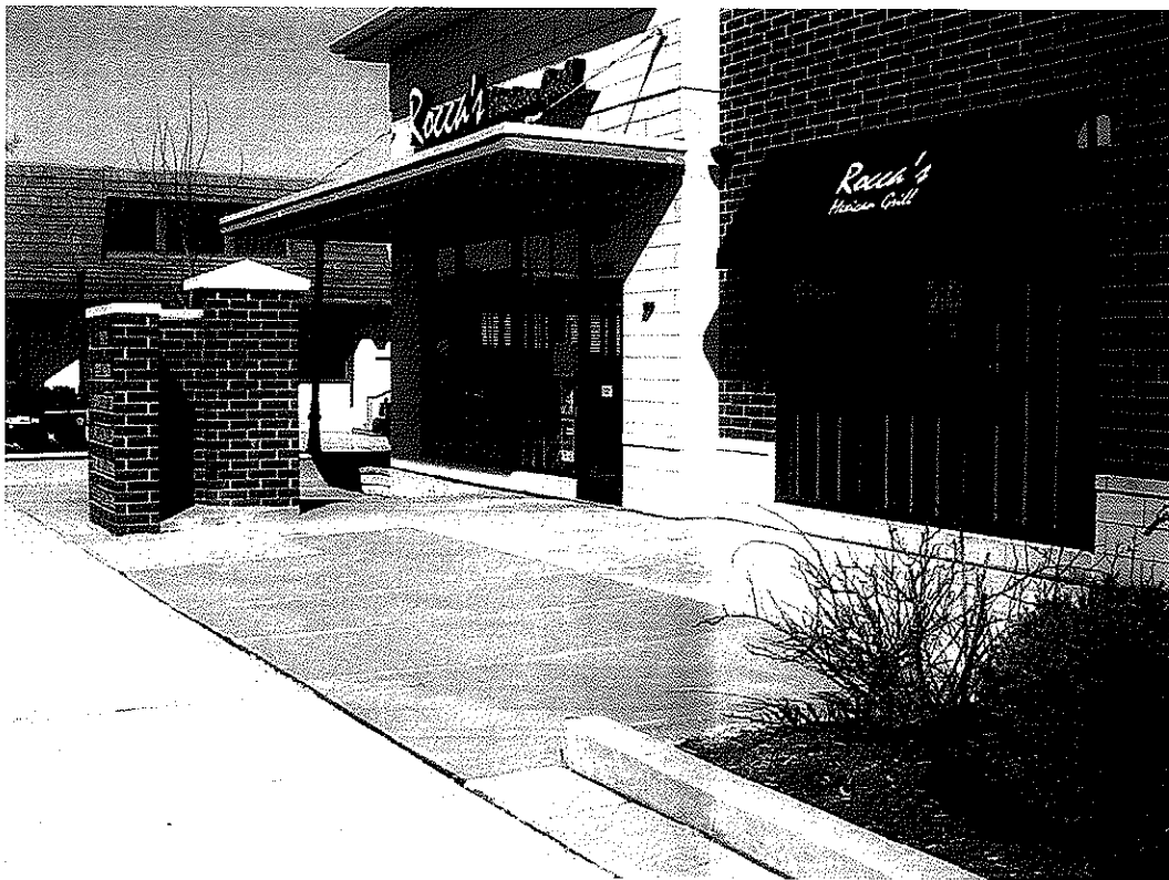
Figure 2 – South seating area looking to the northwest
