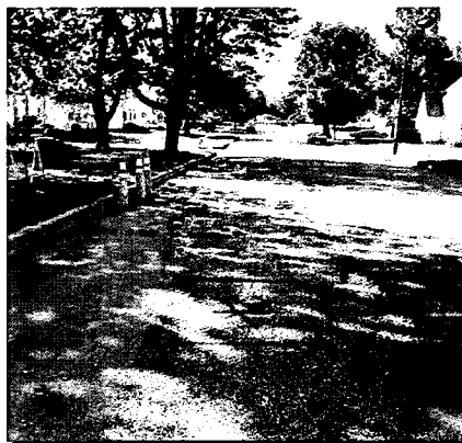
"X" marks the spot for excavation
