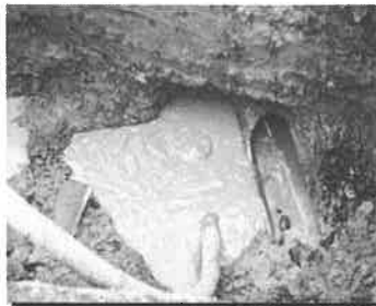
Hidden leak running into drain tile
