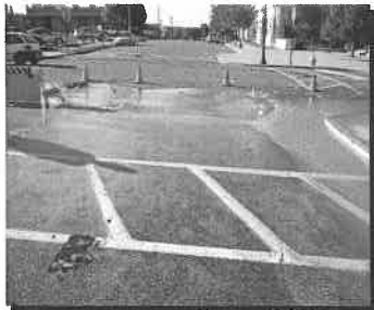
Leak surfacing at intersection
