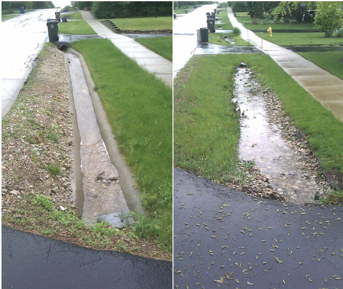
Concrete Line Channel (Left) and Channel Stabilized with Fabric & Rock (Right)
