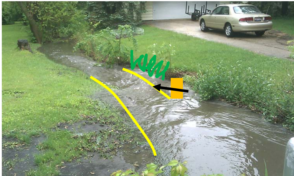
Proposed Sediment Removal & Bendway Weir Deflecting Away from Driveway
