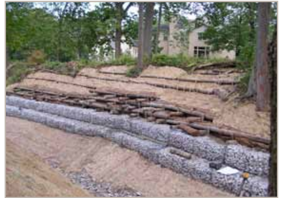
Fort Sheridan Ravine Stabilization, Fort Sheridan, IL
