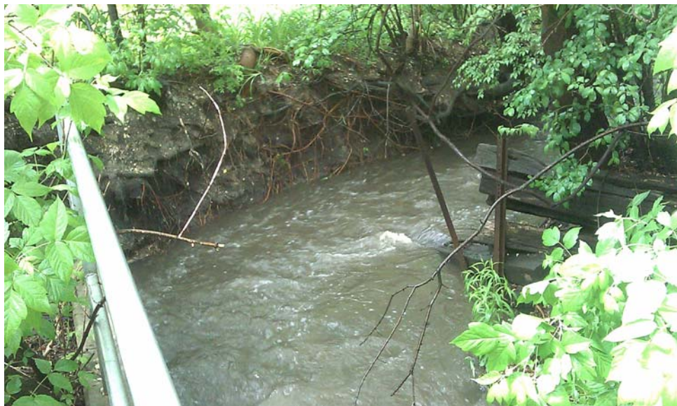
Concrete Wall at Bend Near Washington Street
