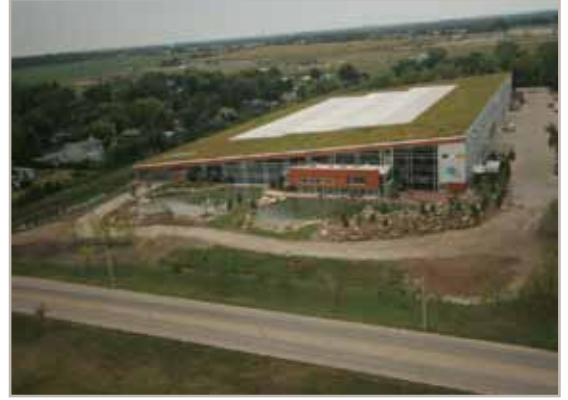
Aquascapes Green Roof, St. Charles, IL
