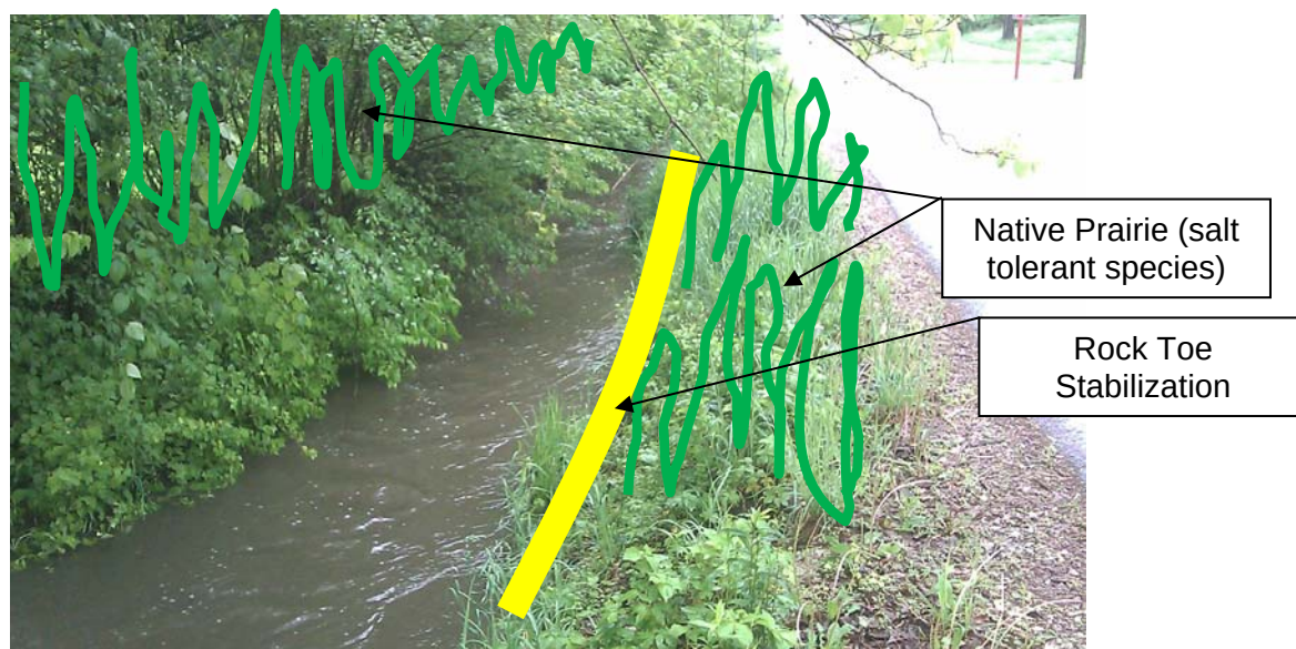
Looking Upstream along Kenyon Street, North Bank in Shade
