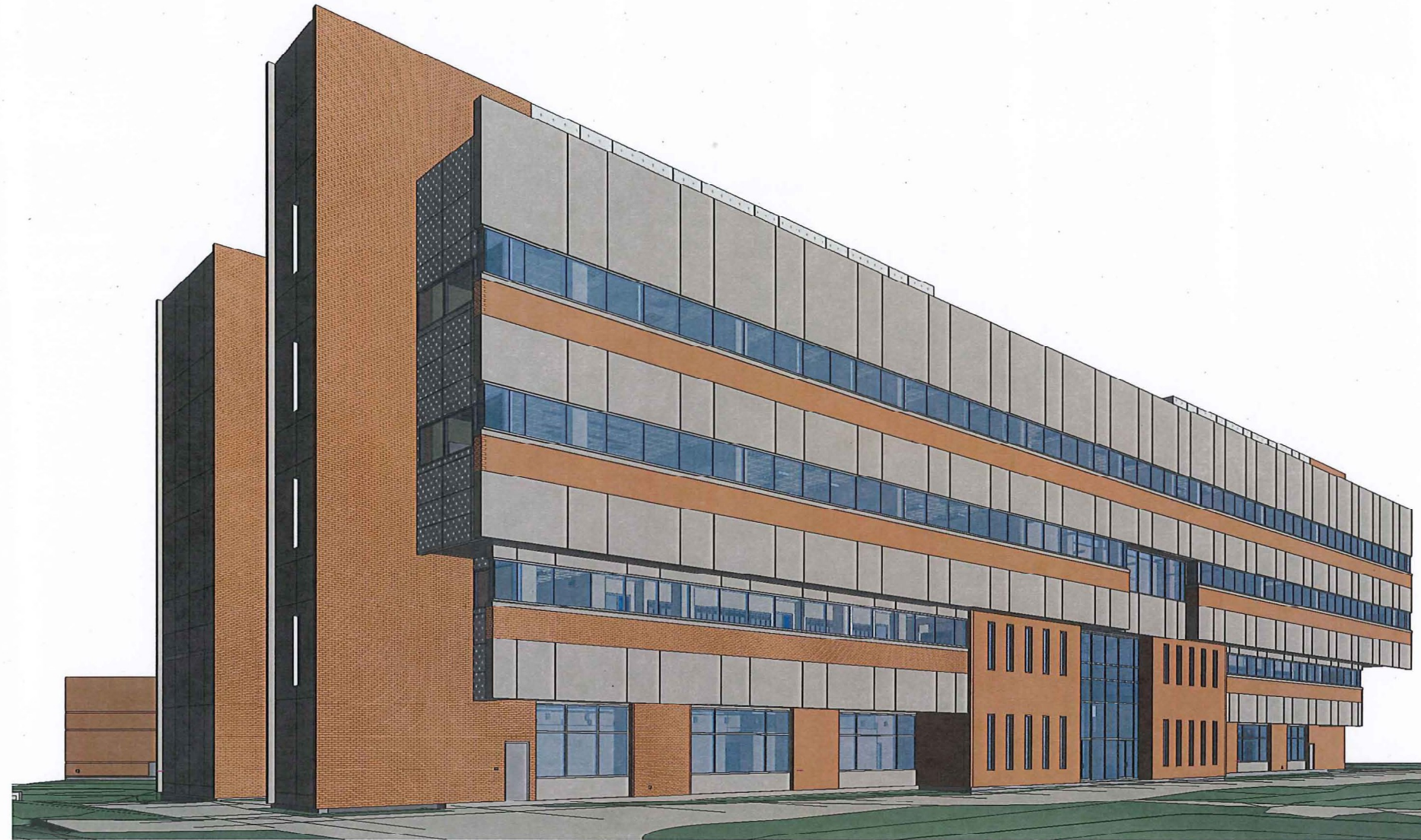
SOUTH EAST VIEW OF BUILDING
