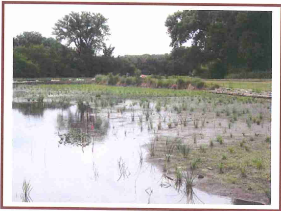
Figure 3: Churchill Woods project in DuPage County – Planting area transition from aquatics to wet meadow.
