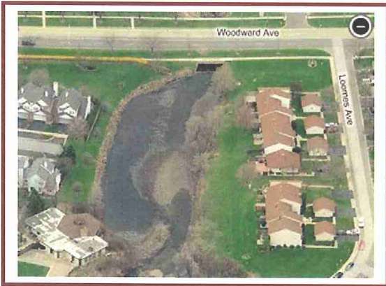
Figure 2: Aerial depicting mud flat and expected open water creek flow
