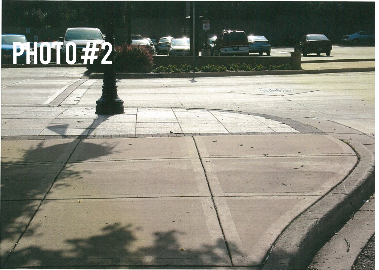
NW corner of Main Street and Grove Street, looking east
