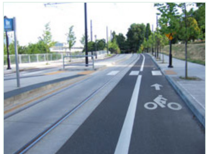
This bike lane has enough width for a bicyclist to comfortably ride between the curb and gutter and the adjacent travel lane.
