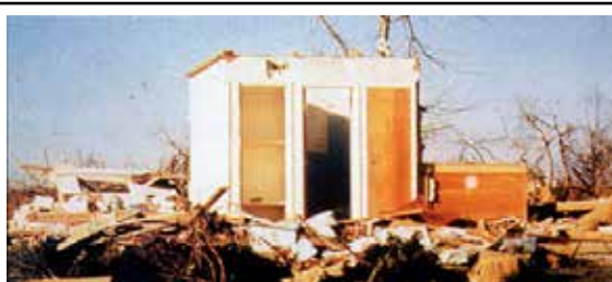
Interior rooms can be reinforced and retrofitted to be tornado “safe rooms”
