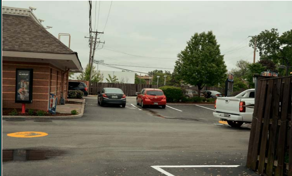
Viewing east through "alleyway" from west property line of McDonald's
