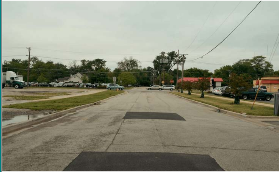
Viewing north along Florence Avenue
