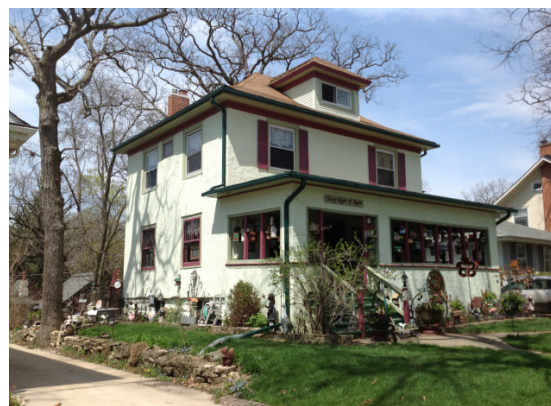
An American Foursquare with some Prairie Style characteristics such as stucco cladding, 4809 Oakwood Avenue, 1920s
