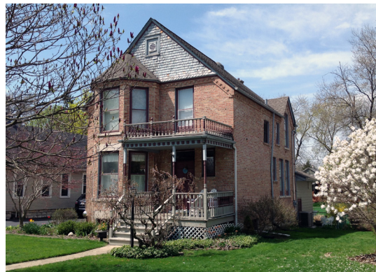
Queen Anne house constructed in brick at 4710 Highland Avenue, 1860s
