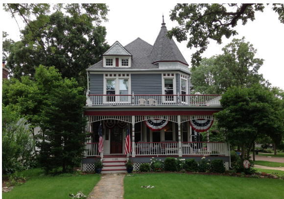
A Queen Anne-styled house with roof tower, 1130 Franklin Avenue, 1890s
