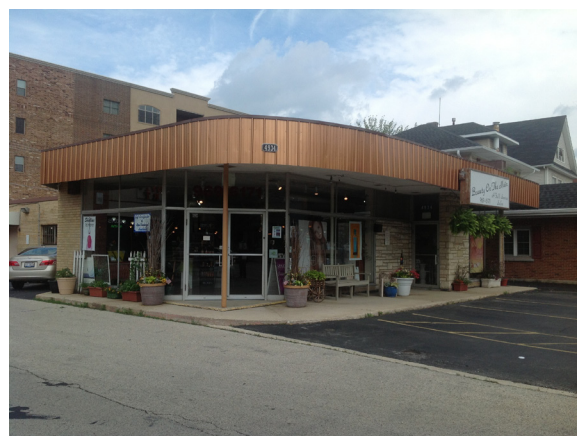
A Strip Commercial building with Mid-Century Modern styling at 4934 Main Street
