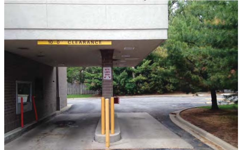
Interior of Drive-Through Area
