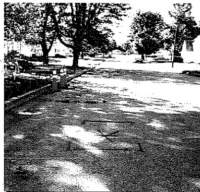
"X" marks the spot for excavation
