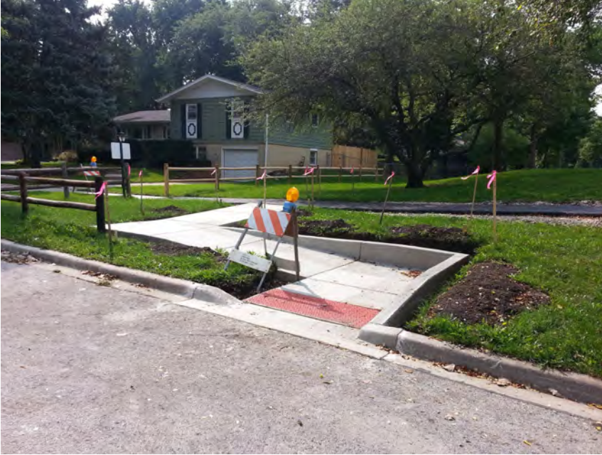
McCollum Park, new accessible entrance on 67th Street
