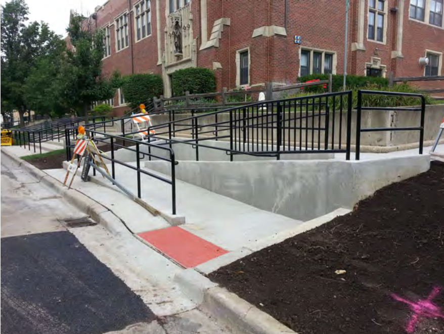
St. Joseph's School, new accessible ramp at Franklin and Highland
