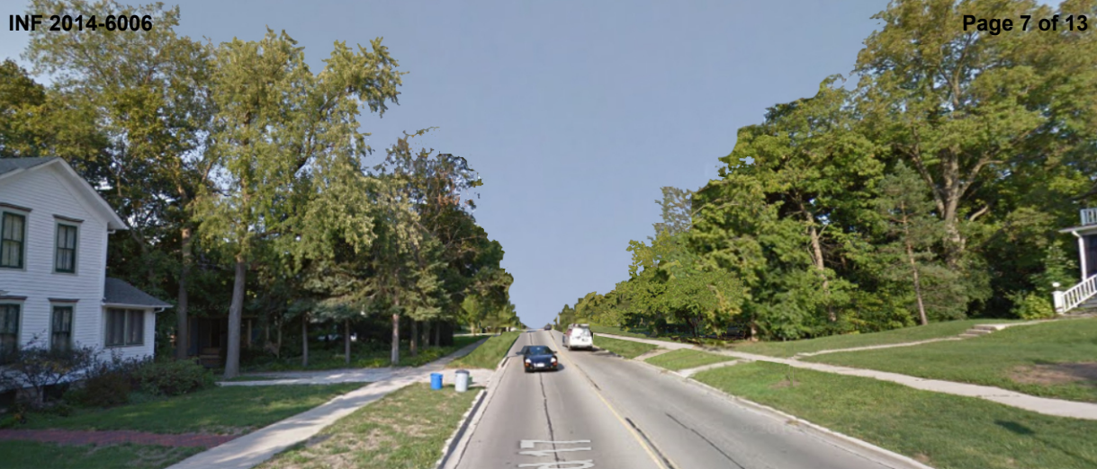
Looking east on Maple Avenue from Lyman Avenue - After tree removal before replanting
