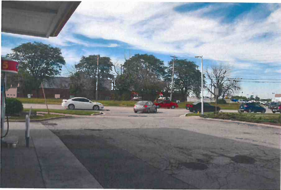
Looking at east drive on Warrenville Rd.
