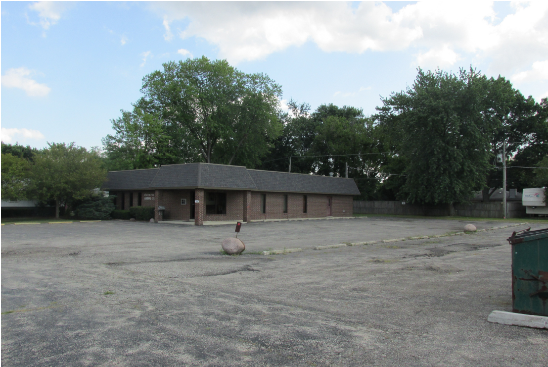
1- Current veterinarian building with a surface parking lot.
