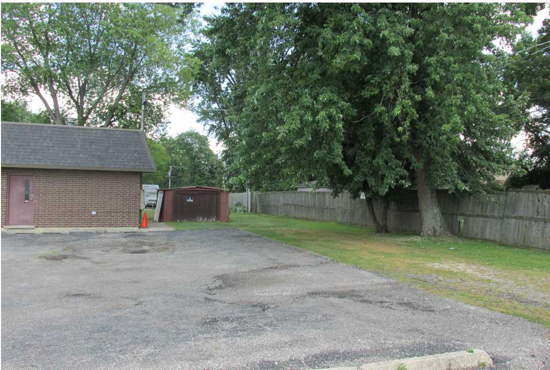
2 Rear of the subject property abutting residential with limited landscaping.
