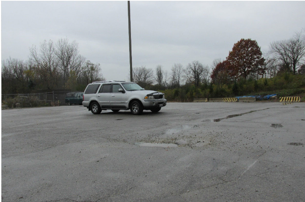
Looking at westernmost property line abutting Lyman Woods.
