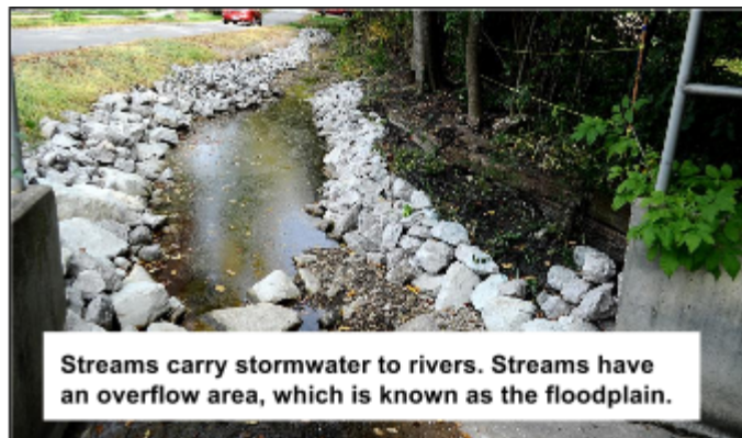
A headwall and culvert allow water to flow under a street
