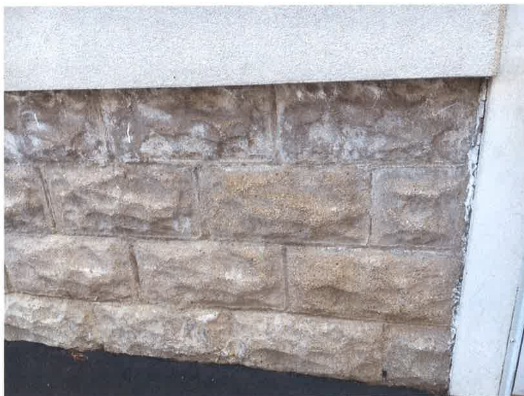
Photo #6: Rusticated concrete block foundation wall – January 10, 2016
