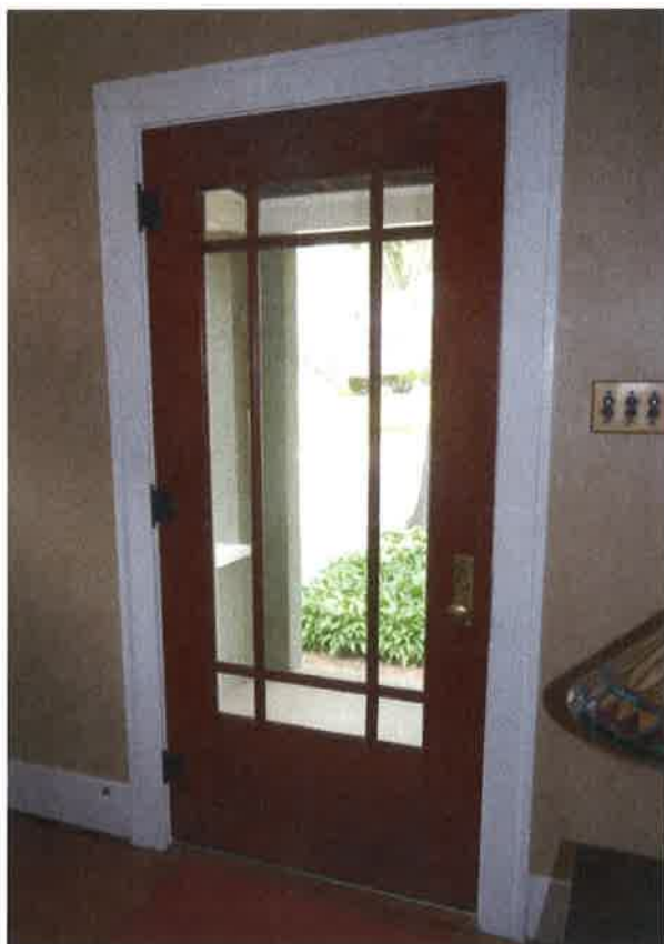
Photo #2: Restored Front door – June, 28, 2015
