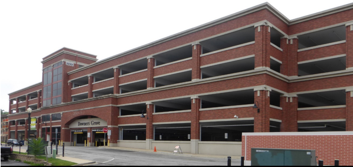
Figure 1- North Elevation of Parking Facility
