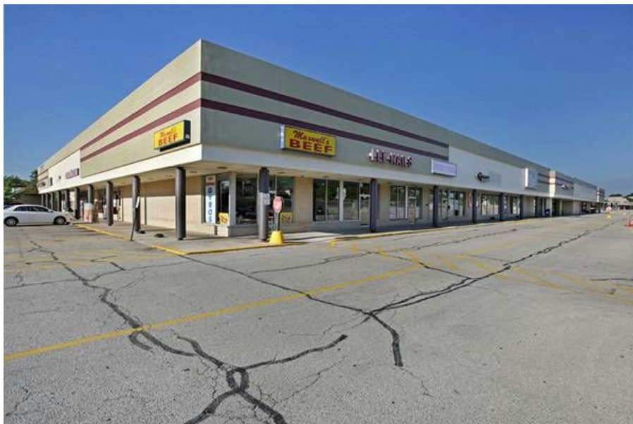
An existing older shopping center in Downers Grove
