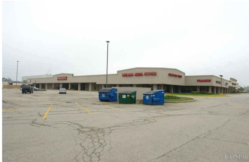
University Plaza on Butterfield Road - a catalyst site identified for retail redevelopment
