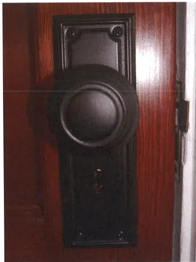
Photo #5: Original door hardware – December 30, 2015
