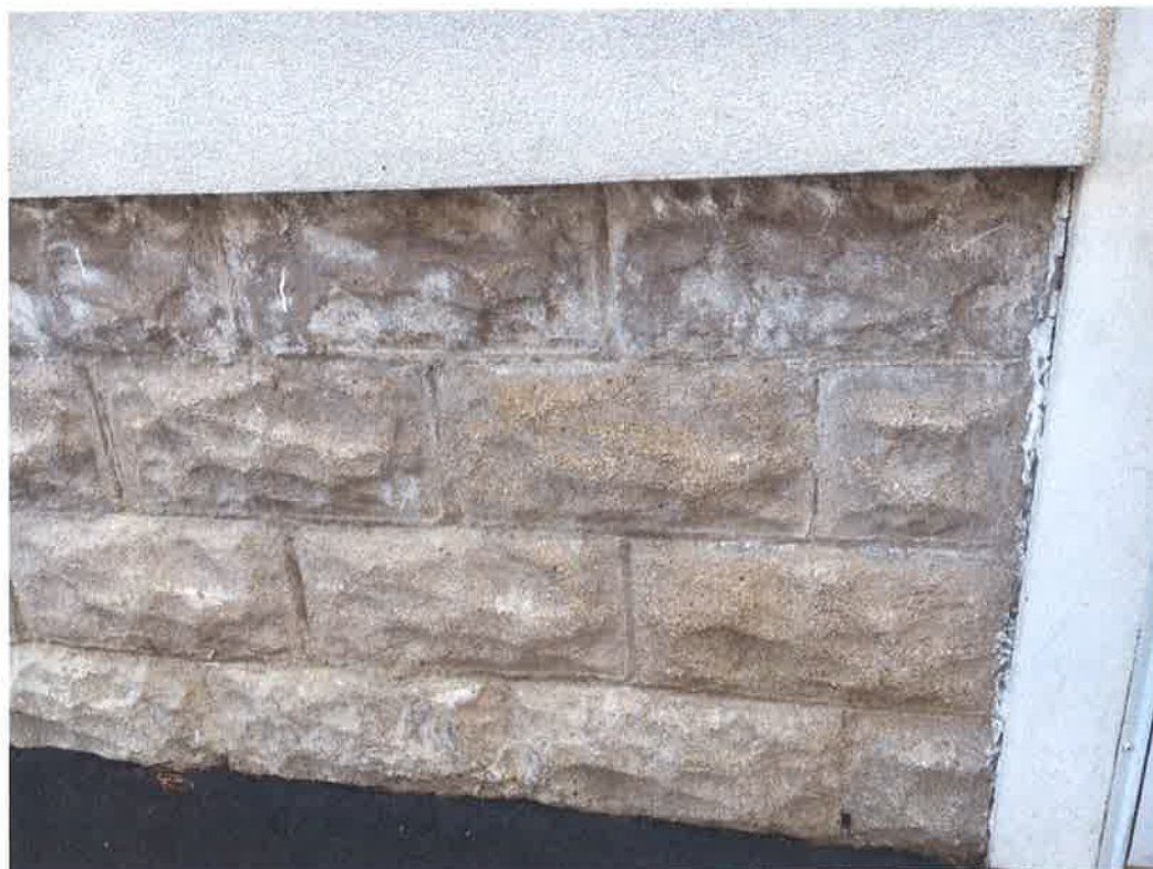
Photo #6: Rusticated concrete block foundation wall – January 10, 2016
