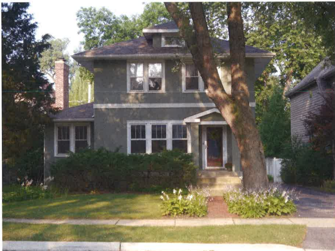
Photo #1: Front (East) Elevation - September 3, 2015
