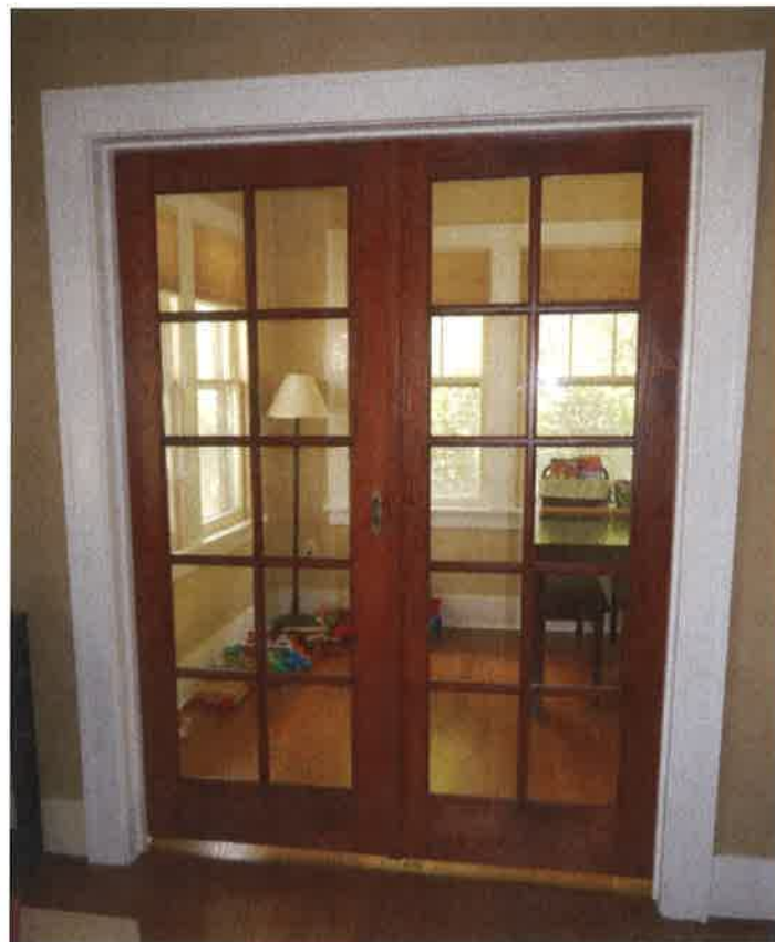
Photo #3: Restored Sunroom French doors– June 28, 2015
