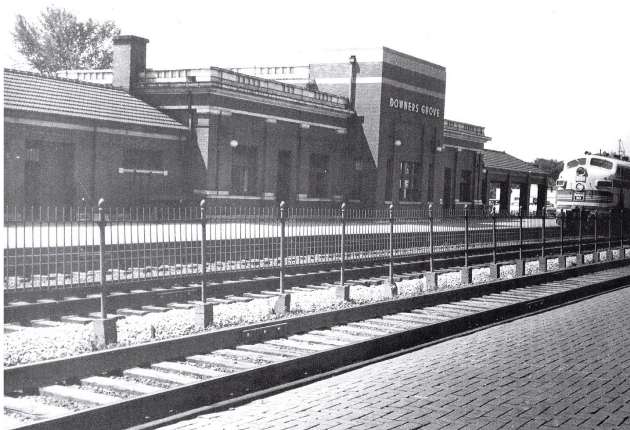
Photo #4 View looking southwest – 1955
