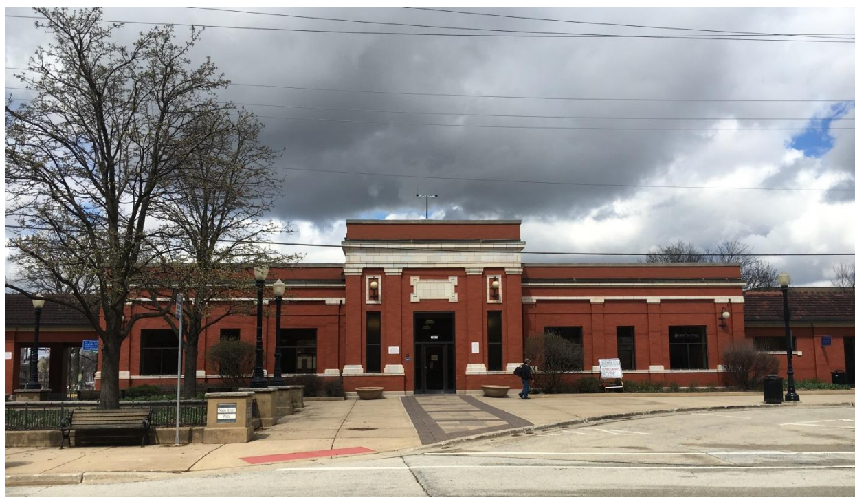
Photo #12 Main building south elevation
