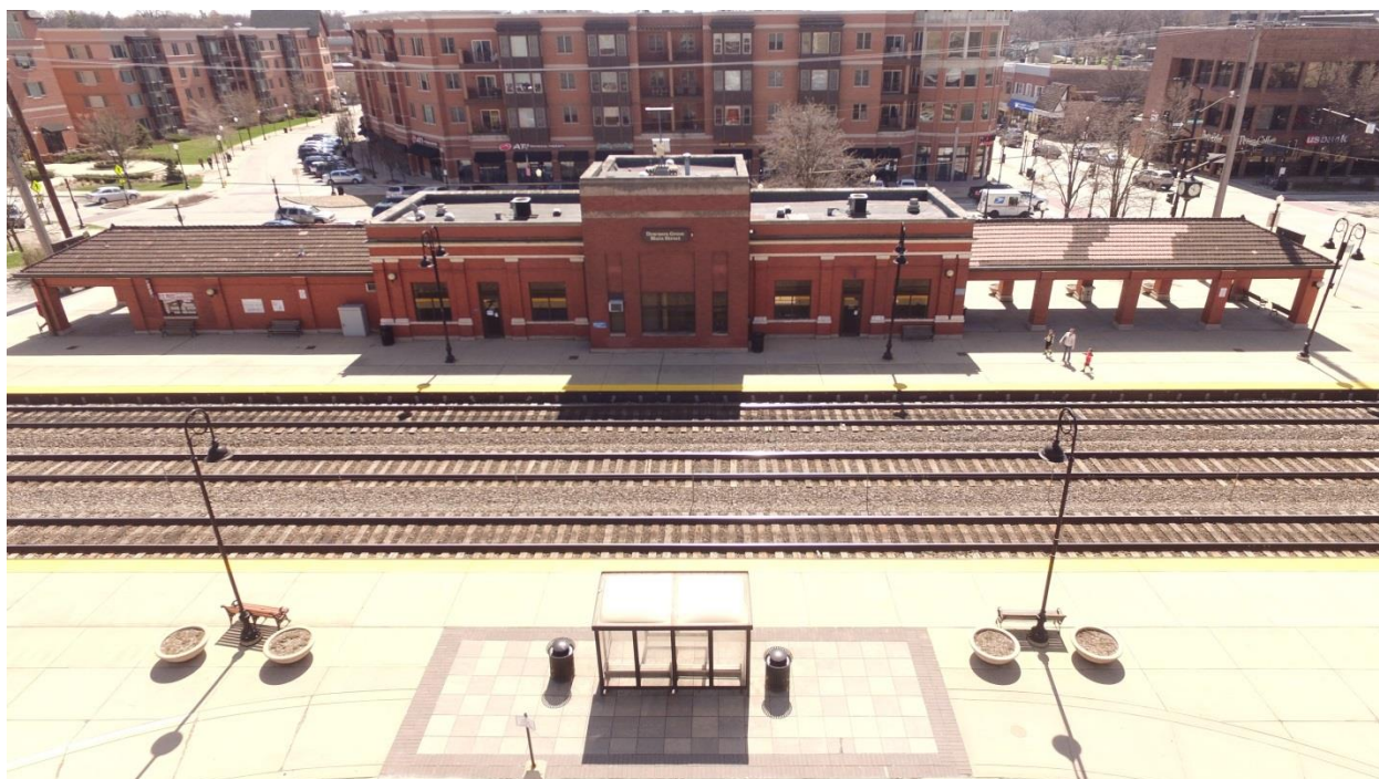
Photo #10 North elevation
