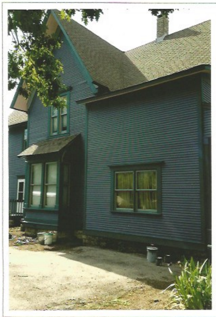
Photo #5: South view
