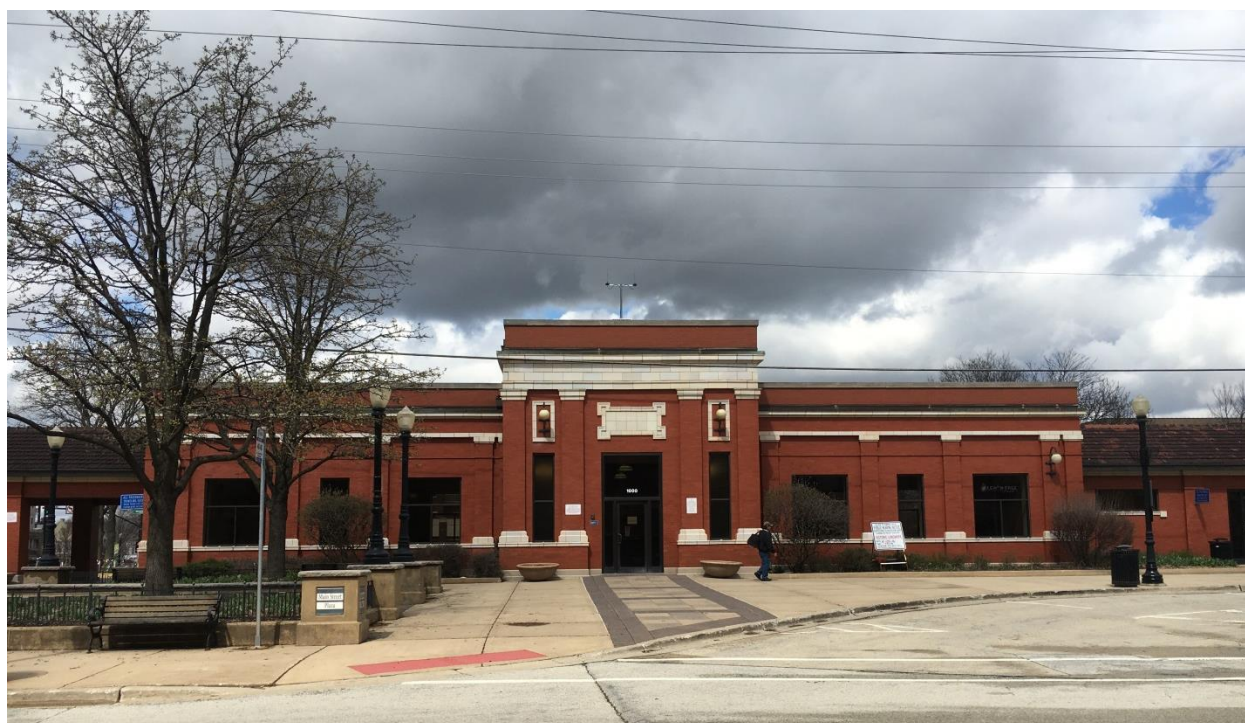
Photo #12 Main building south elevation
