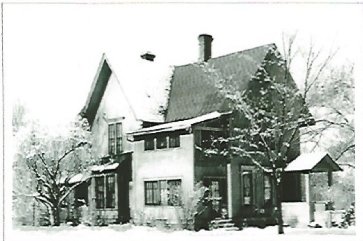
Photo #1: 5226 Carpenter Street circa 1940
