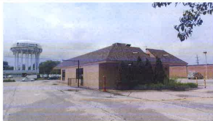
EXISTING LANDSCAPING AT BACK OF BUILDING
