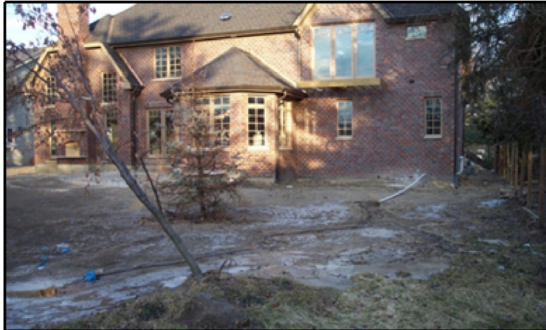
Runoff from sump pumps
