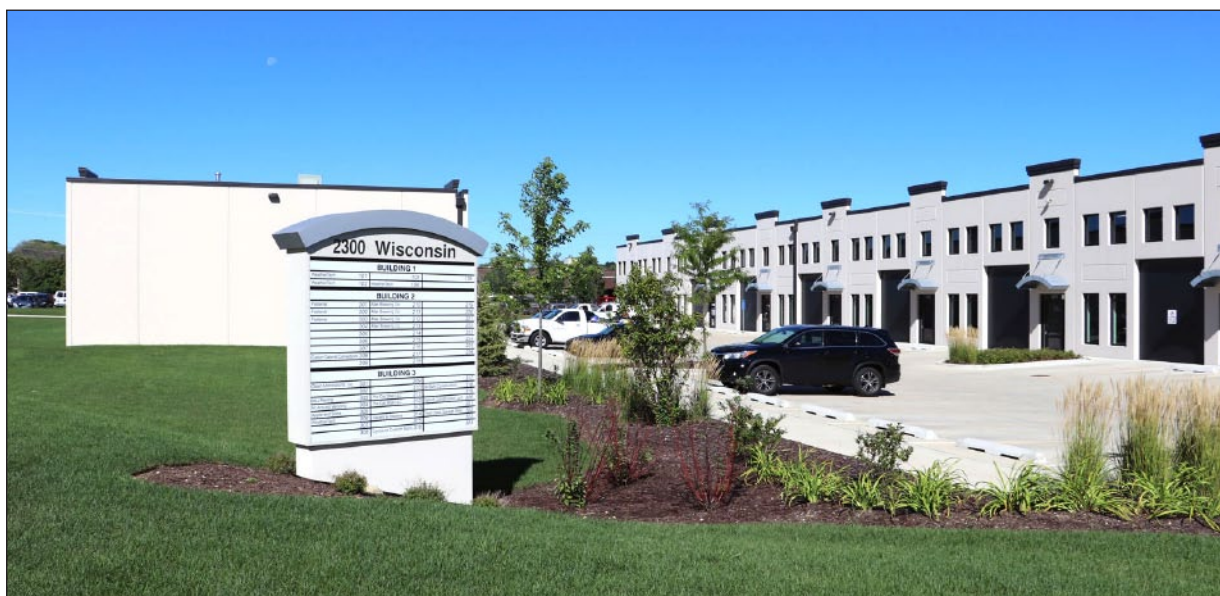
Subject Property - View Looking West from Driveway
