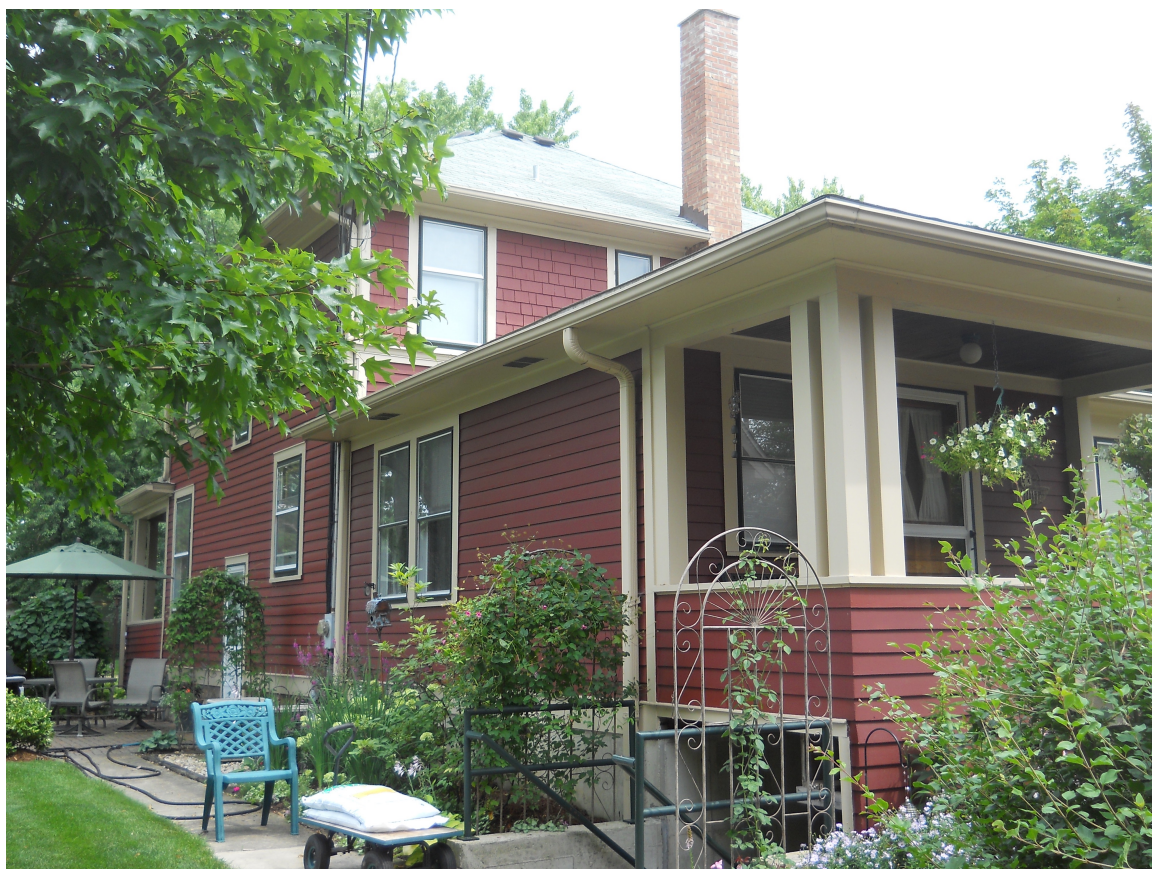
Photo #9 West View of addition porch with triple columns – August 30 2016
