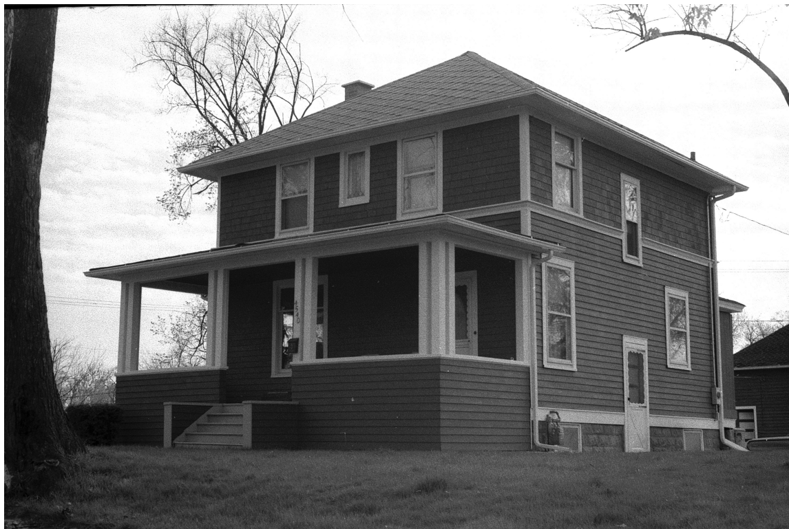
Photo #3 View from NE – March 1981
