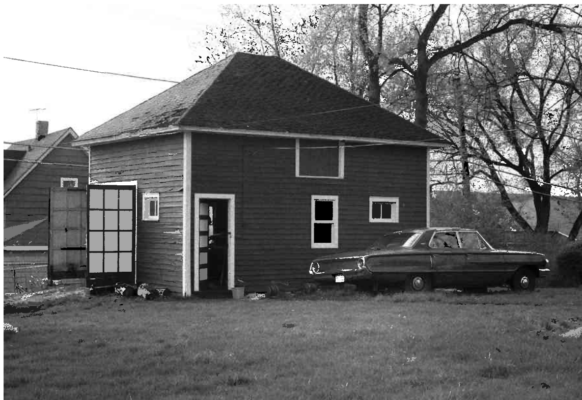
Photo # 5 Carriage House – March 1981
