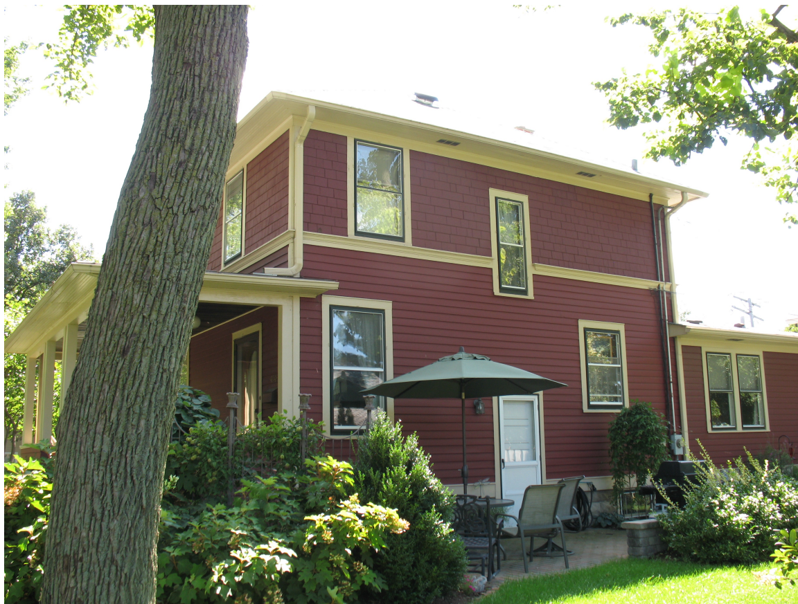
Photo #8 NE View – August 30, 2016
