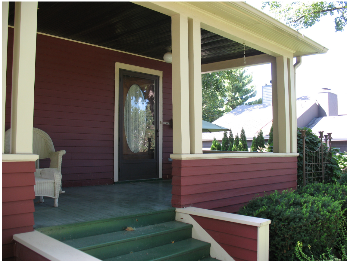
Photo #10 Front porch, detail of columns and front door with oval glass – August 30, 2016
