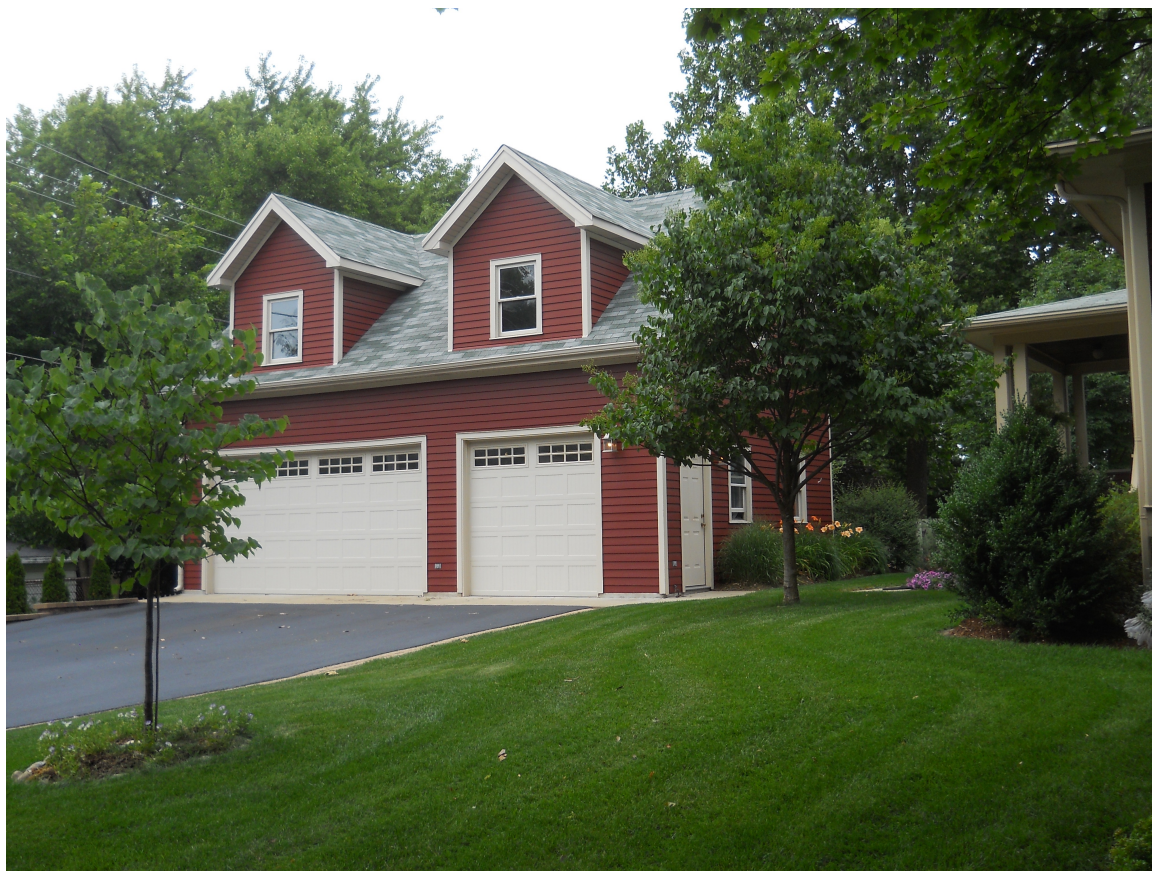
Photo #11 Garage built 2006 – August 30, 2016
