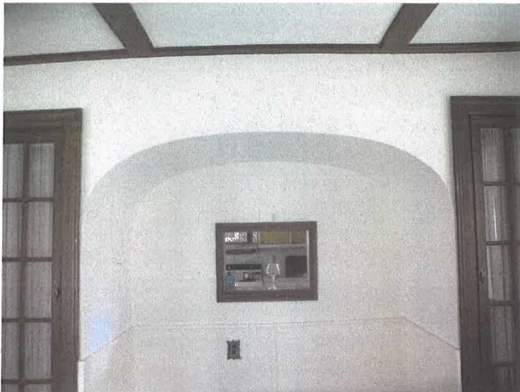
Photo #5: Dining room arch and kitchen pass-through: side cabinets and ceiling beams partially visible (2016)
