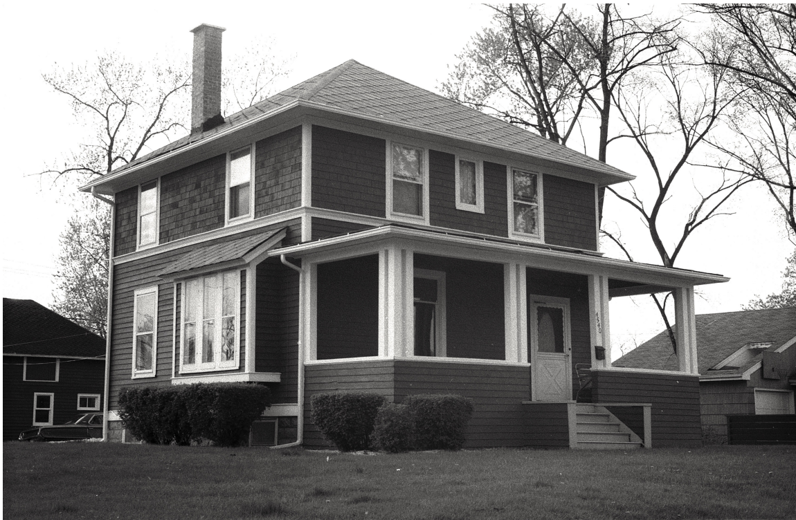
Photo #2 View from SE - March 1981
