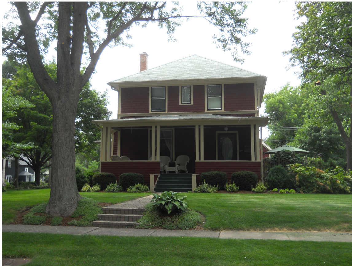
Photo #6 East Elevation – August 30, 2016
