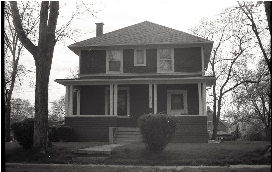
Photo #1 East elevation - March 1981
