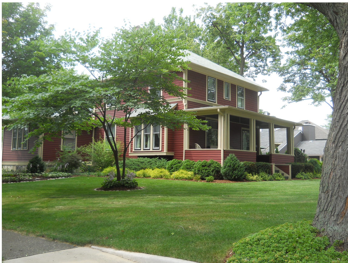
Photo #7 SE View – August 30, 2016
