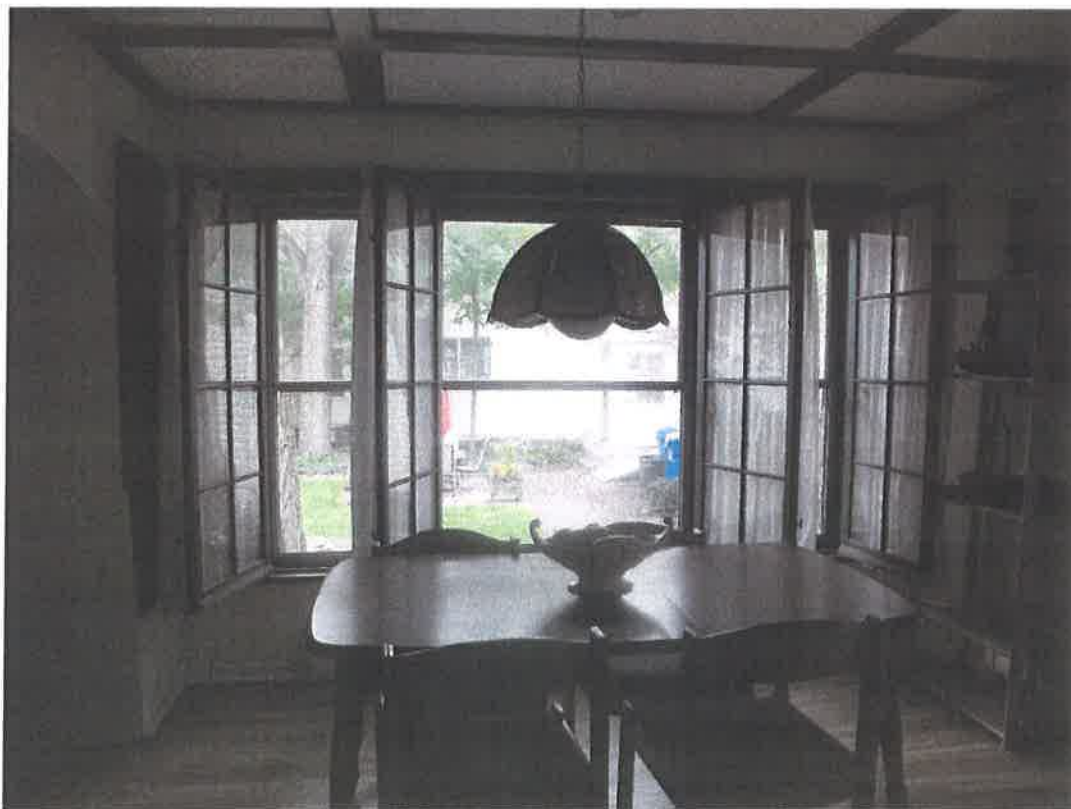
Photo #6: Casement windows on dining room east wall
