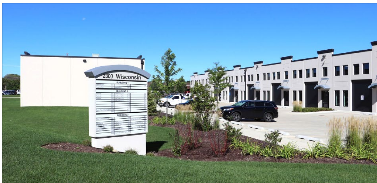
Subject Property - View Looking West from Driveway
