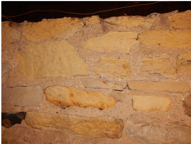
Original stone and mortar upper basement wall foundation
