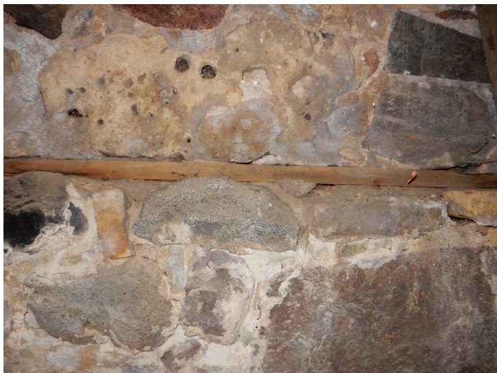
Original larger boulders at base of foundation
