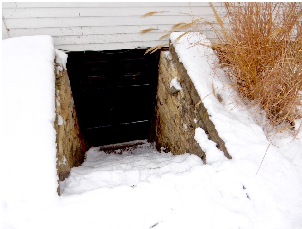
Original stone steps to exterior basement entrance. This entrance was used to provide safe haven for escaping slaves as part of the Underground Railroad during the Civil War era.
