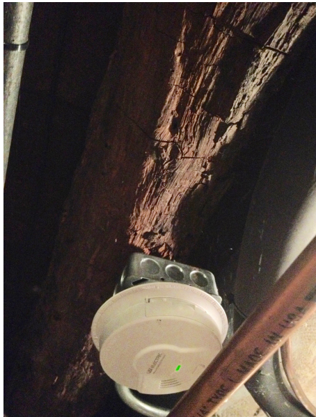
1840s hand-hewn timber joist in basement with present-day smoke and fire alarm
