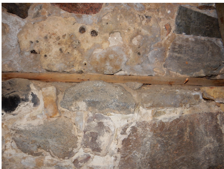
Original larger boulders at base of foundation
