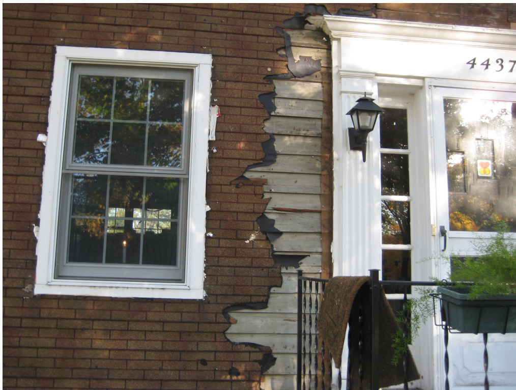
Close up showing original clapboard covered with 1930's brown, fake-brick tar paper after aluminum siding removed (photographed during 2008 exterior residing project)
