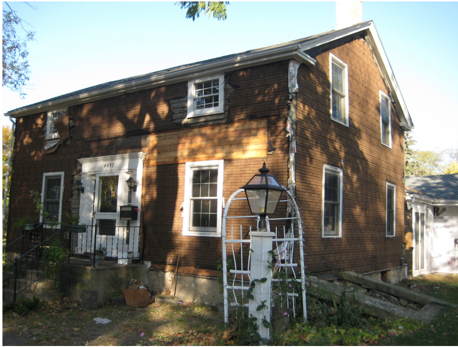
House after removal of 1960's vintage 8-inch aluminum siding and prior to installation of 4-inch fiber-cement siding (photographed during 2008 exterior residing project)
