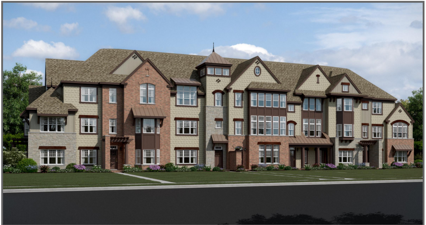
Similar project under construction in Libertyville
