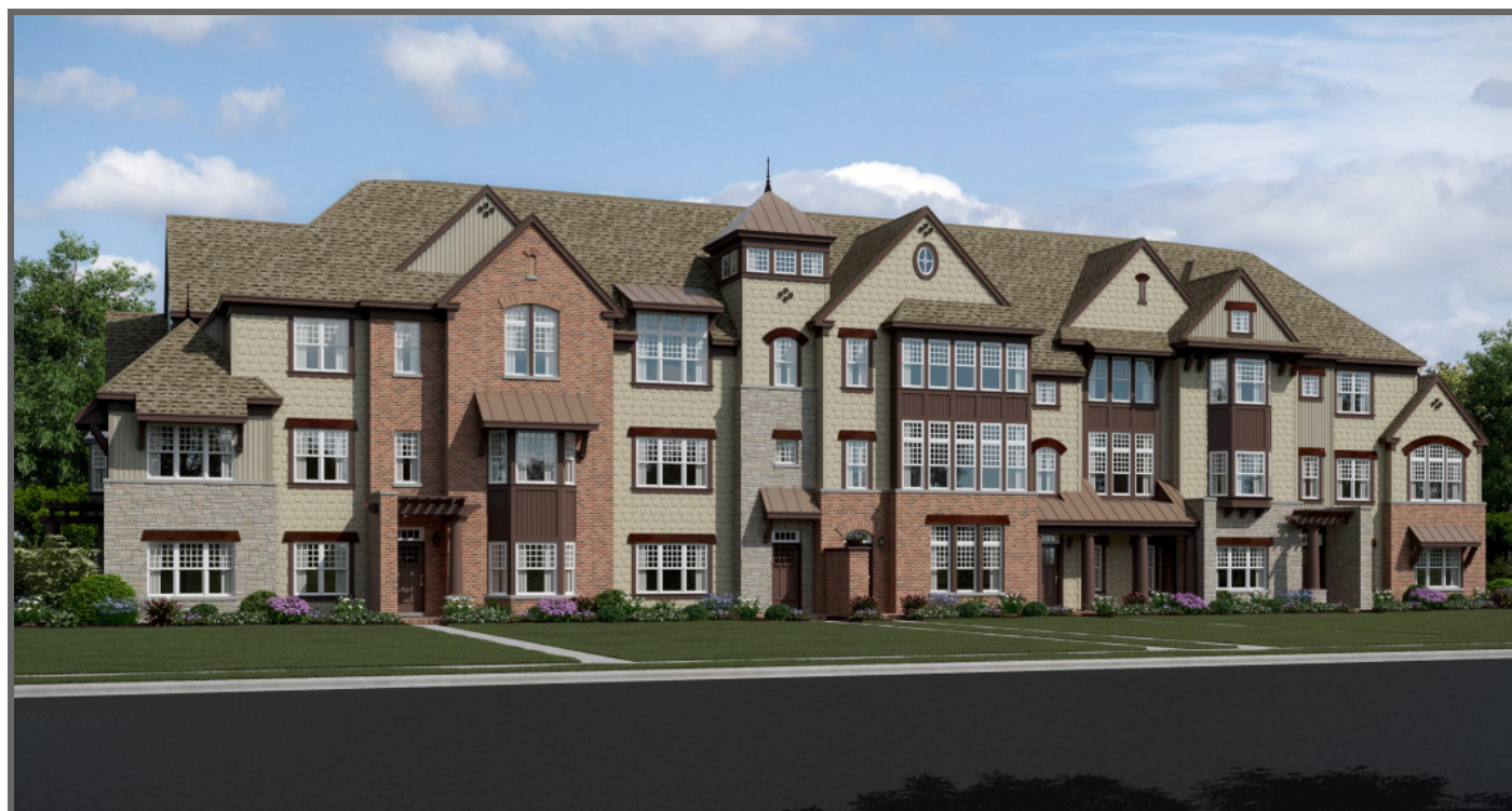
Similar project under construction in Libertyville
