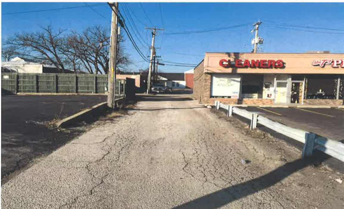
VIEW WEST ALONG THE SUBJECT ALLEY
