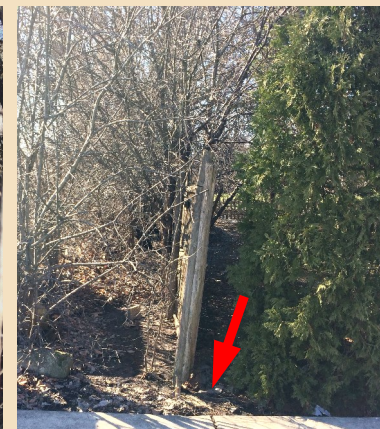
2 Outfall from LPDA 101
