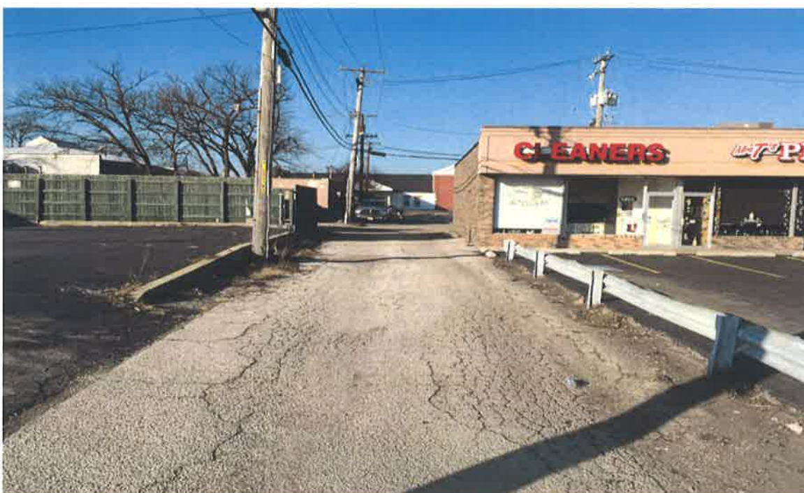
VIEW WEST ALONG THE SUBJECT ALLEY
